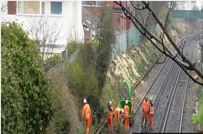
Clearance of trees on track embankment
